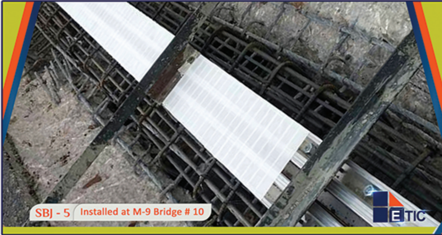
SBJ - 5 Installed at M-9 Bridge # 08
