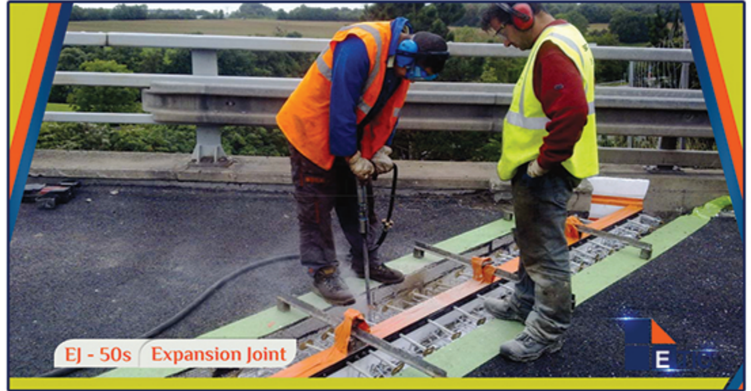
EJ - 50s Has Been Installed at Koral Chowk Islamabad Express Highway.
