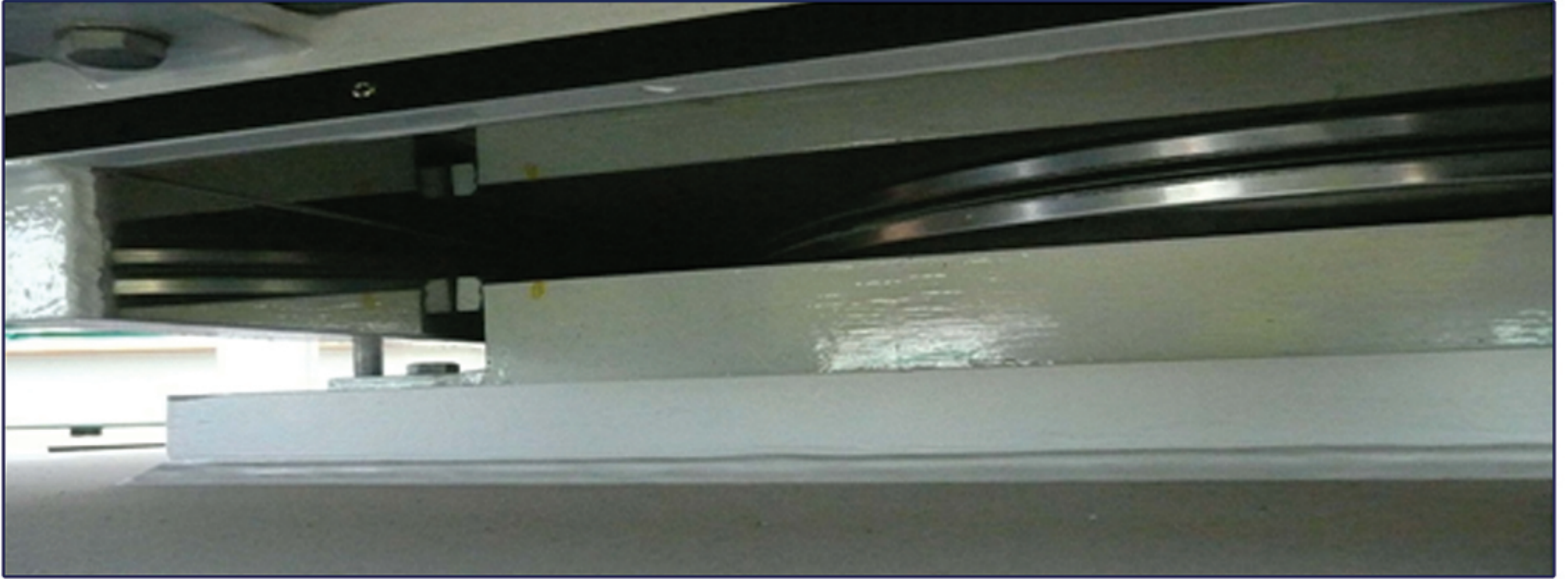
Installed 7500 tons injectable pot-bearings
