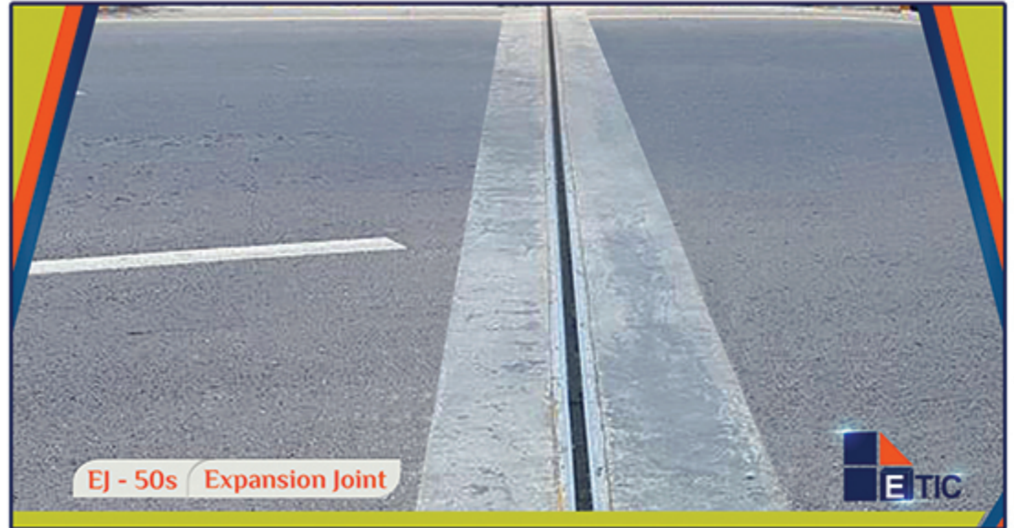
EJ - 50s Has Been Installed at Koral Chowk Islamabad Express Highway.
