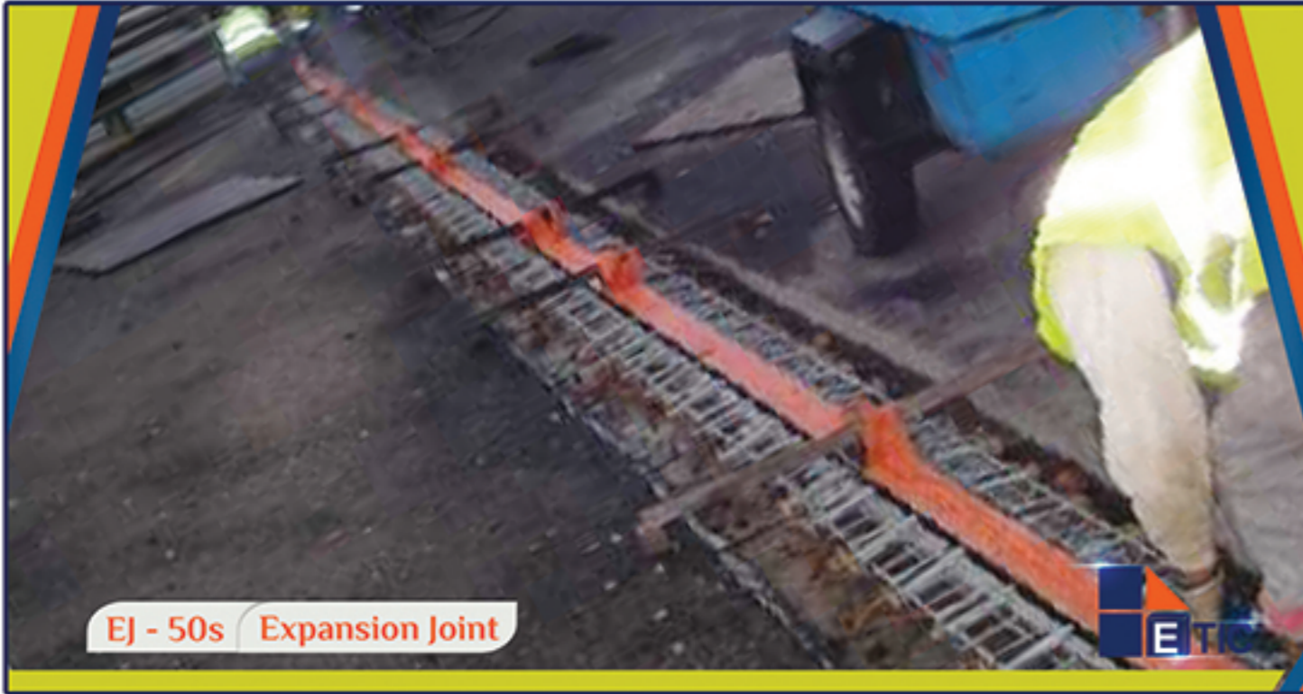
EJ - 50s Has Been Installed at Koral Chowk Islamabad Express Highway.
